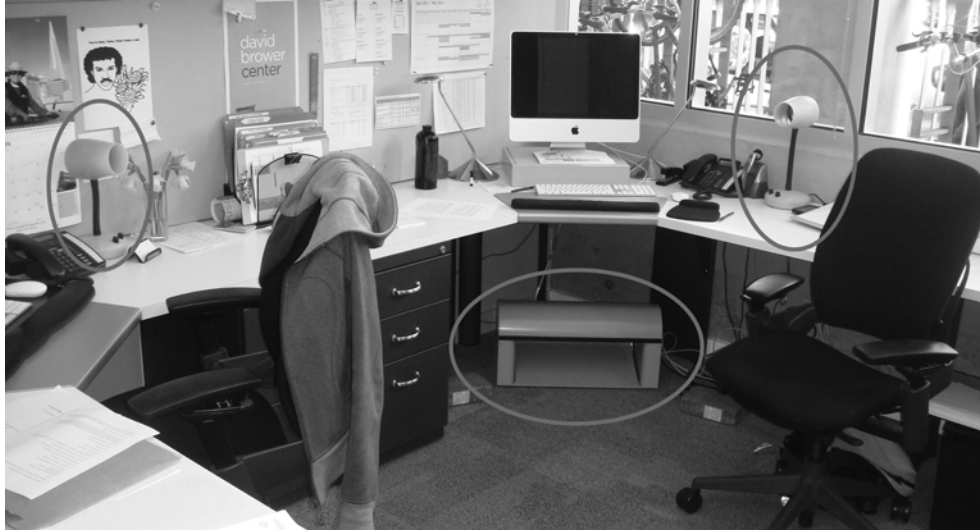
Figure H.6 Personal Environmental Control Devices (Fans and a Radiant Foot Warmer) in an Office Photograph by Ed Arens (Courtesy of Center for the Built Environment).
